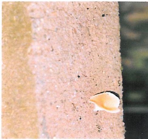
Wood Cement composite building block also grew fungal growth. Fungal growths (Peziza Genus)
