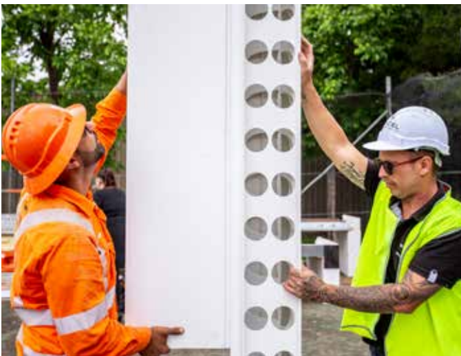
8: Install 1 to 2 main profiles (P-1) on both sides of the corner.
