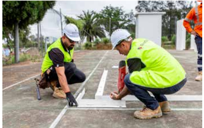
4: Place angles on at least one face of the corner, where:
