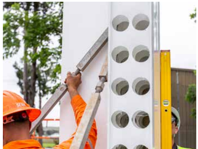
11: Plumb assembled corner through the use of diagonal braces.
