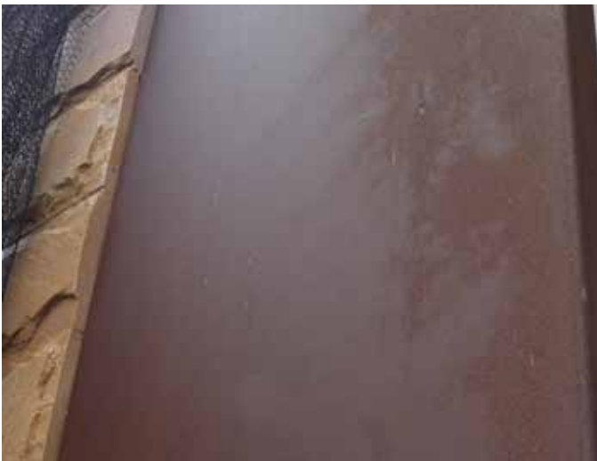
Weathered 'Corten' steel cladding
