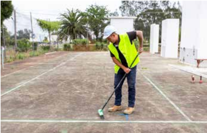
1: Clean substrate ready for set out.
