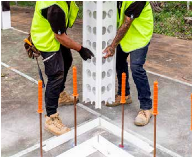
Where applicable, start the wall installation with a corner profile (P-5).
