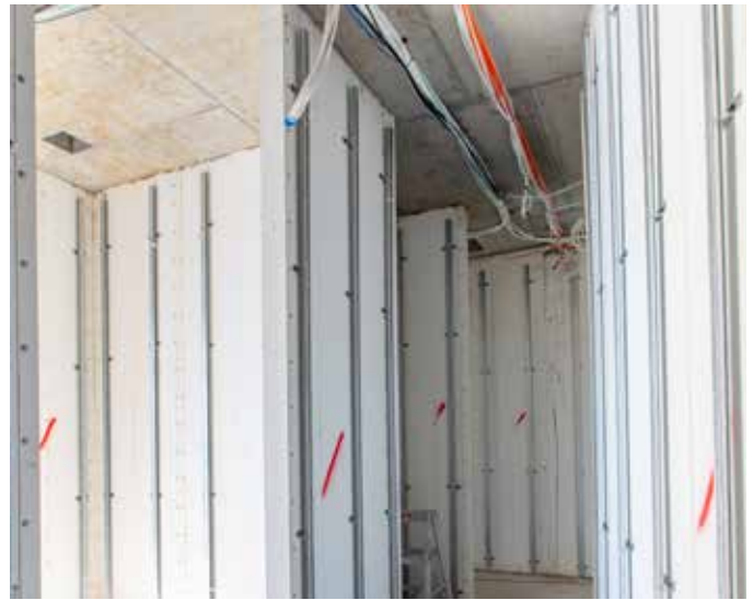
Example of furring channel attachment onto Dincel walling
