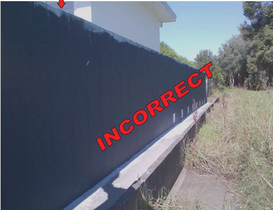
WESTERN FENCE WALL – AFTER RENDER
