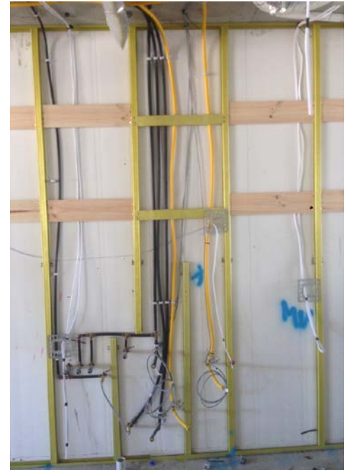
Internal Walls Fitted with Services Structural Work – Service Trade Coordination
