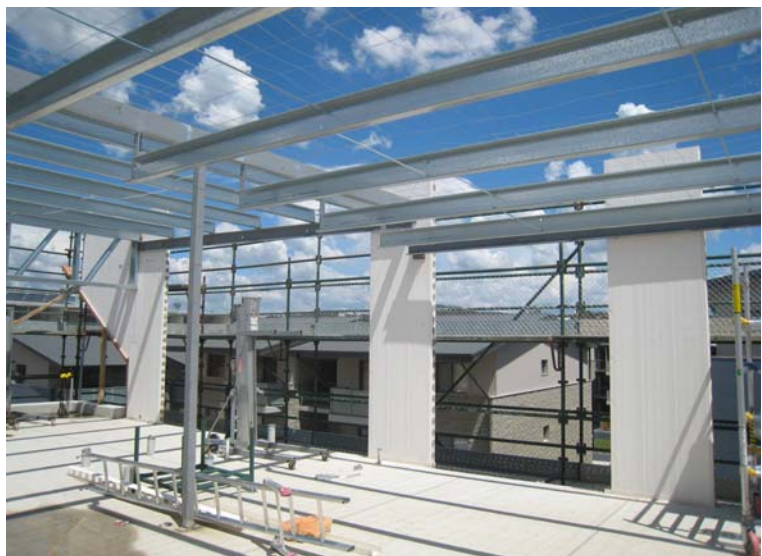
Dintel Columns Supporting Roof
