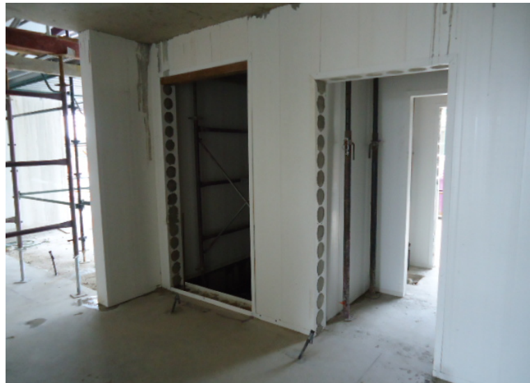
Dintel Lift and Stair Shaft Walls
