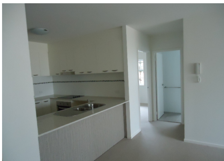
Plasterboard Finished Internal Dintel Walls
