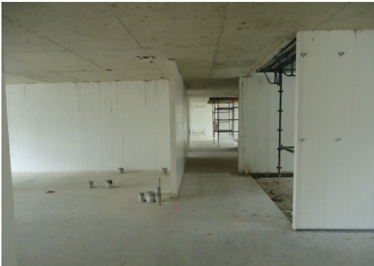
Internal Loadbearing Unreinforced 110mm Dintel Walls
