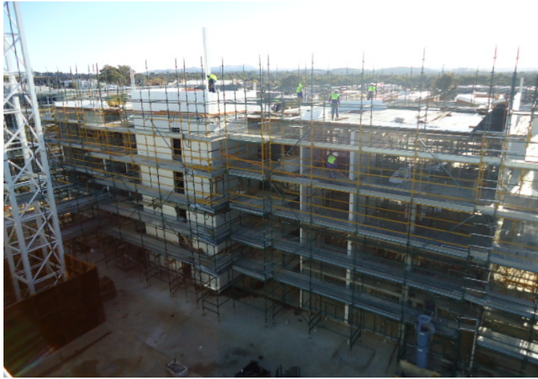
Loadbearing Dintel Walls
