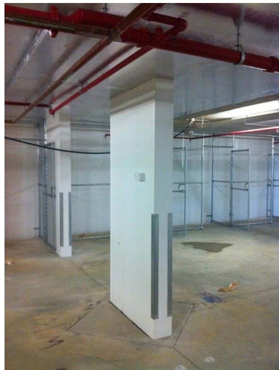
Dintel Basement Columns and Walls
