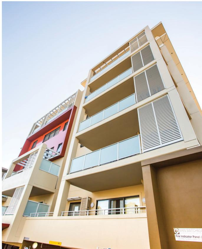
The Dincel Wall applications include 200 Dincel Wall for retaining walls, fire corridor walls, lift shaft walls and stair shaft walls. 110 Dincel Walls were adopted for all apartment inter-tenancy party and corridor walls and 200 Dincel Walls were adopted for all external facade walls.
